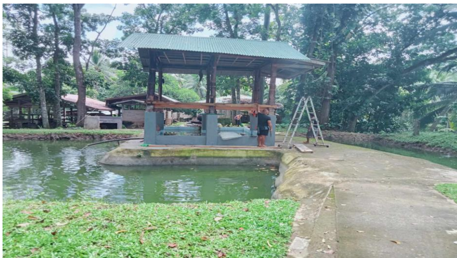
New building constructed after the old one was demolished
