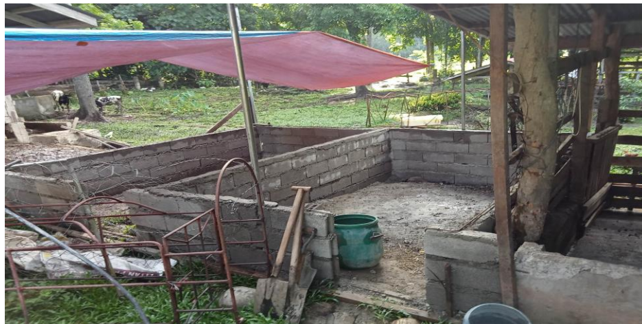
Pig pen undergoing repair
