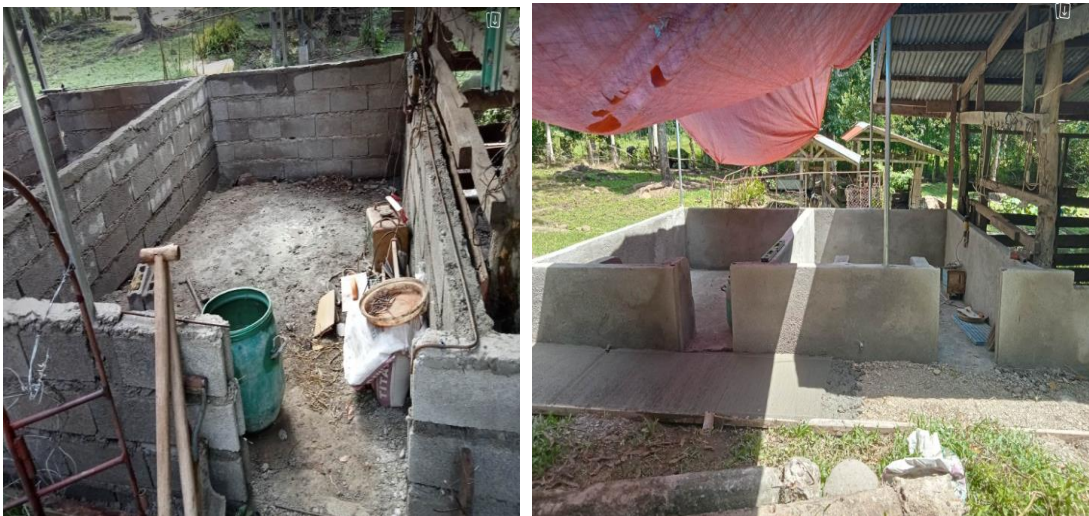
Pig pens under repair
