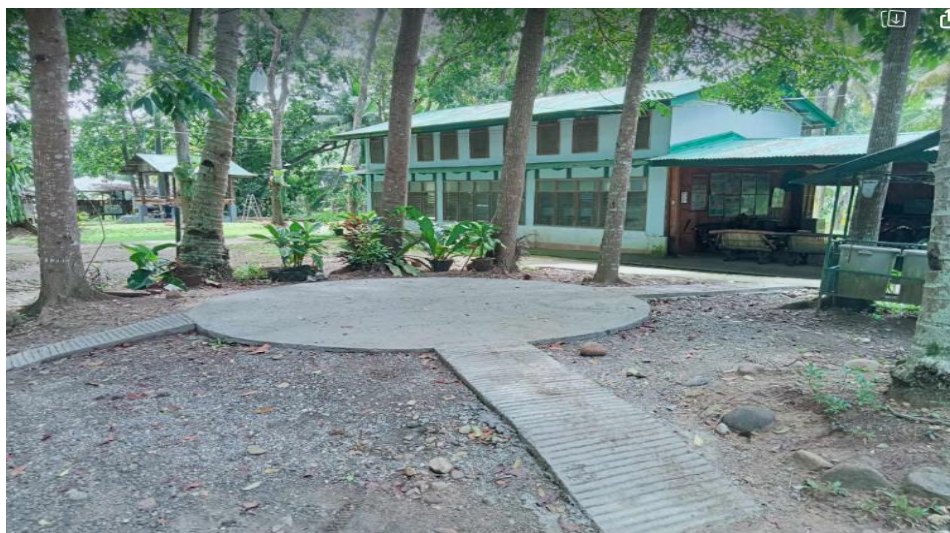
Pathways/walkways are cemented
