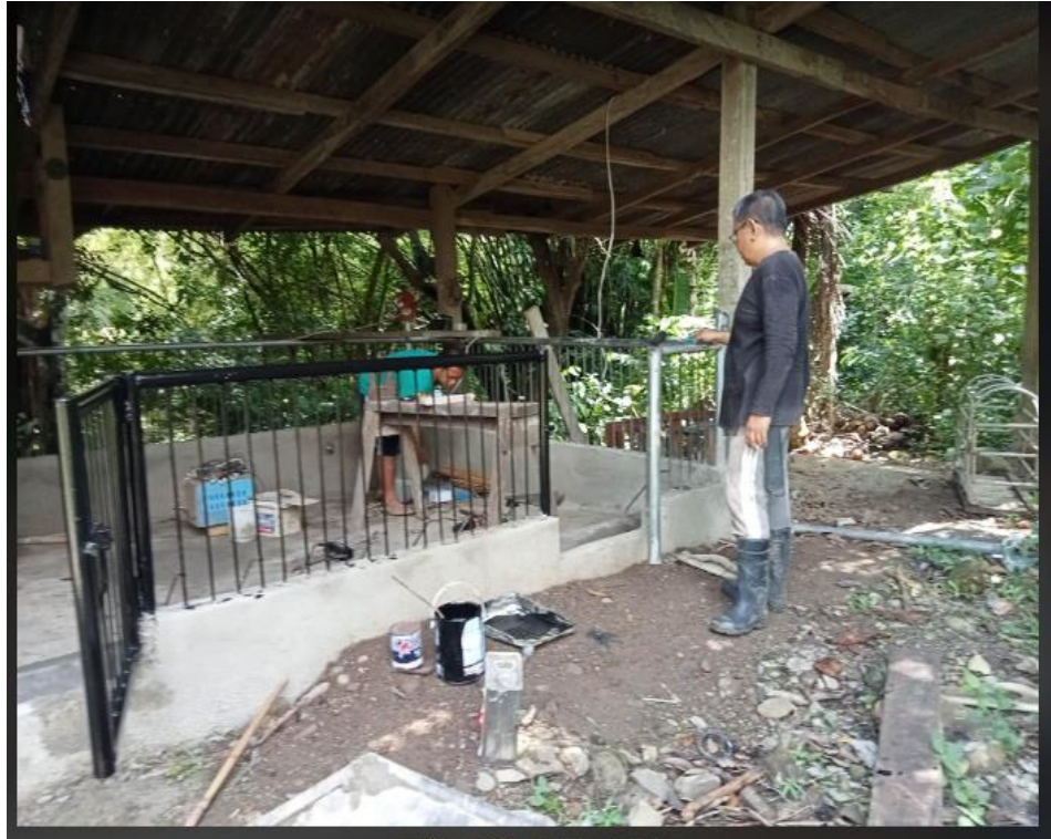
Pig pens were repaired using concrete materials and iron bars.
