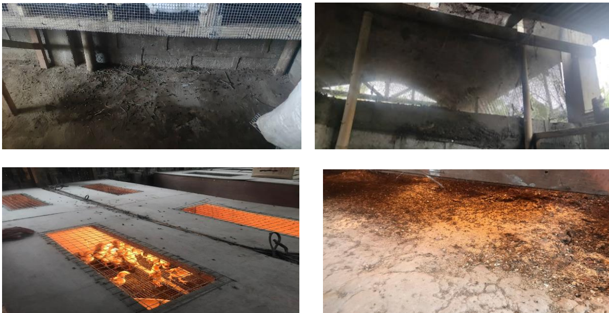
Figure 1. A major problem on housing ventilation and sanitation was observed.
