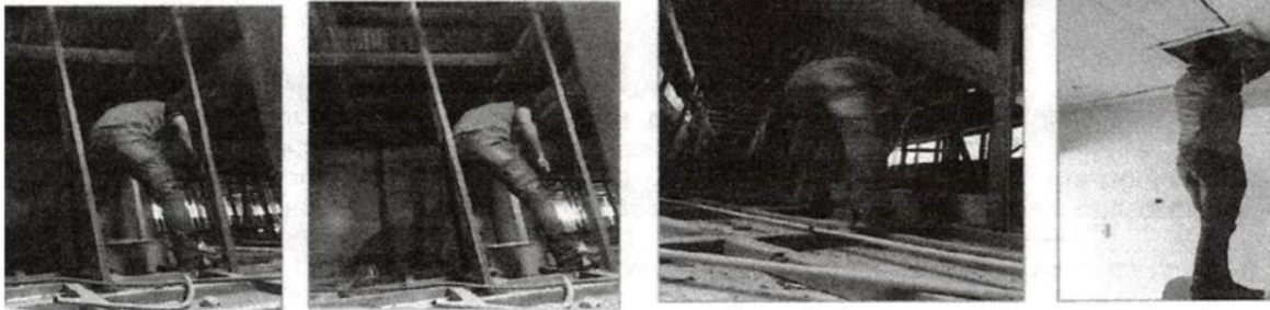
Inspection and treatment at ceiling area for possible termites' infestation.
